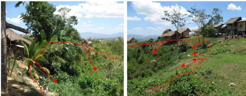
**Figure 6 Residential Houses in Barangay Pange constructed near the headgully of an ephemeralcreek. This is susceptible to landslide during, intense rainfall**
